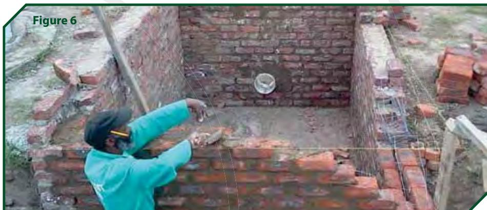
Figure 6: A local builder constructing an 8m<sup>3</sup> biogas digester at the University of Fort Hare, Alice campus, this is part of job creation at local level. The builder was trained by scientists at the Fort Hare Institute of Technology to construct digesters (source: University of FortHare).
